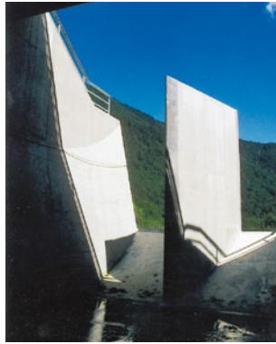
Figure 2a: New spillway: ski-jump of the new spillway
