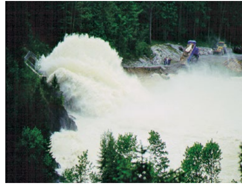
Figure 2b: New spillway: first use of the new spillway with 260 m 3 /s over the ski-jump on 23 May 1999
