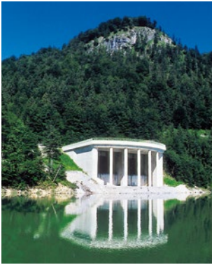
Figure 1: Intake structure for the new spillway
